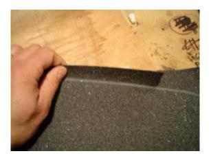
**18]** Next, quickly fold up the excess grip tape along the edge of the deck. This will make it easy to cut.
