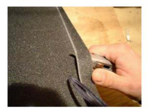
**20]** The deck will be your guide and will hold the razor blade in place as you move around its outline. Be careful when cutting by the wheel wells, and around the edges. If you make any mistakes, they can be fixed later.
