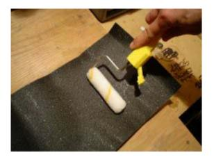
7] If you have a small paint roller, roll down the middle of the deck, making sure there are no air bubbles in the grip tape. Note: if there are any air bubbles left in the grip tape after you have rolled the entire deck, then you can use your razor blade to puncture the grip tape at that spot. Then just press down until all of the air has escaped.
