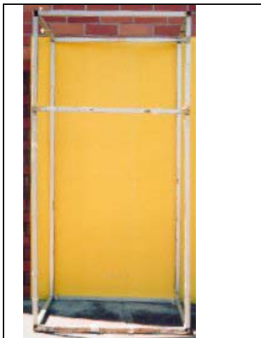
Frame. The front bar supports the proscenium.
